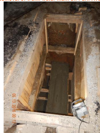
16" sewer replacement on Park Ave W between E 42 nd St and E 41 st St
