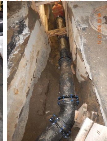
Installation of 12" water main on E 42 nd St between Park and Vanderbilt Aves
