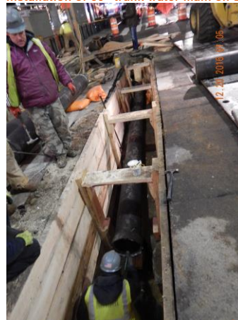
Installation of 12" water main on E 42 nd St between Park and Vanderbilt Aves
