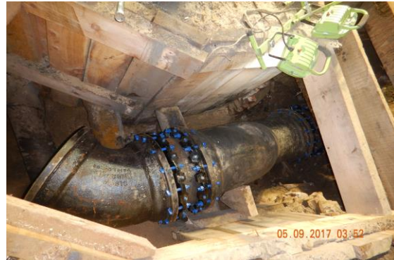
20" Outlet Connection on E 42 St between Park & Lexington Aves.
