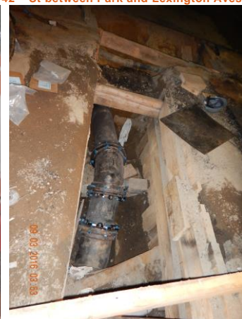
Installation of 12" water main on Park Ave West between E 41 st and E 40 th Sts
