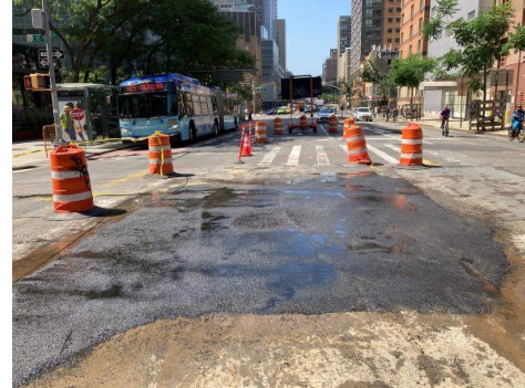
Completed Test Pit at E. 35 th St. @1 st Ave.
