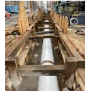
Trunk Water Main Installation- 3 rd Ave bet E 33 rd & E 34 th St
