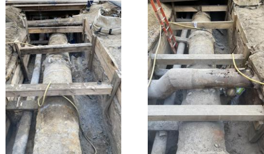
Utility Work on East 35 th Street @ 1 st Avenue
