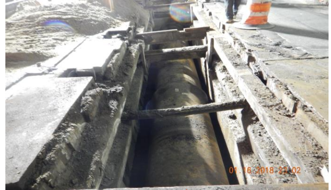
Installation of 36" trunk water main on E 40 th St btwn Park & Madison Aves.
