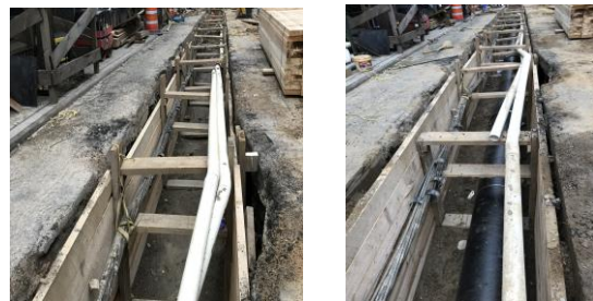
20" Distribution Water Main installation E. 33 rd St. bet 2 nd & 3 rd Ave's.
