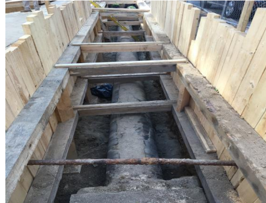
Existing utility steam main in preparation to be removed and replaced
