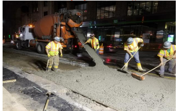
Concrete base placement on E 42 St between Park & Lexington Aves.
