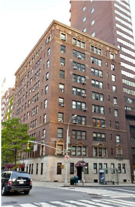
Madison Avenue side
